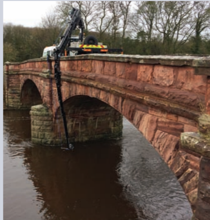
Bridgecat in action (above) and sonar image (below) showing cross-section between river bank and bridge abutment
